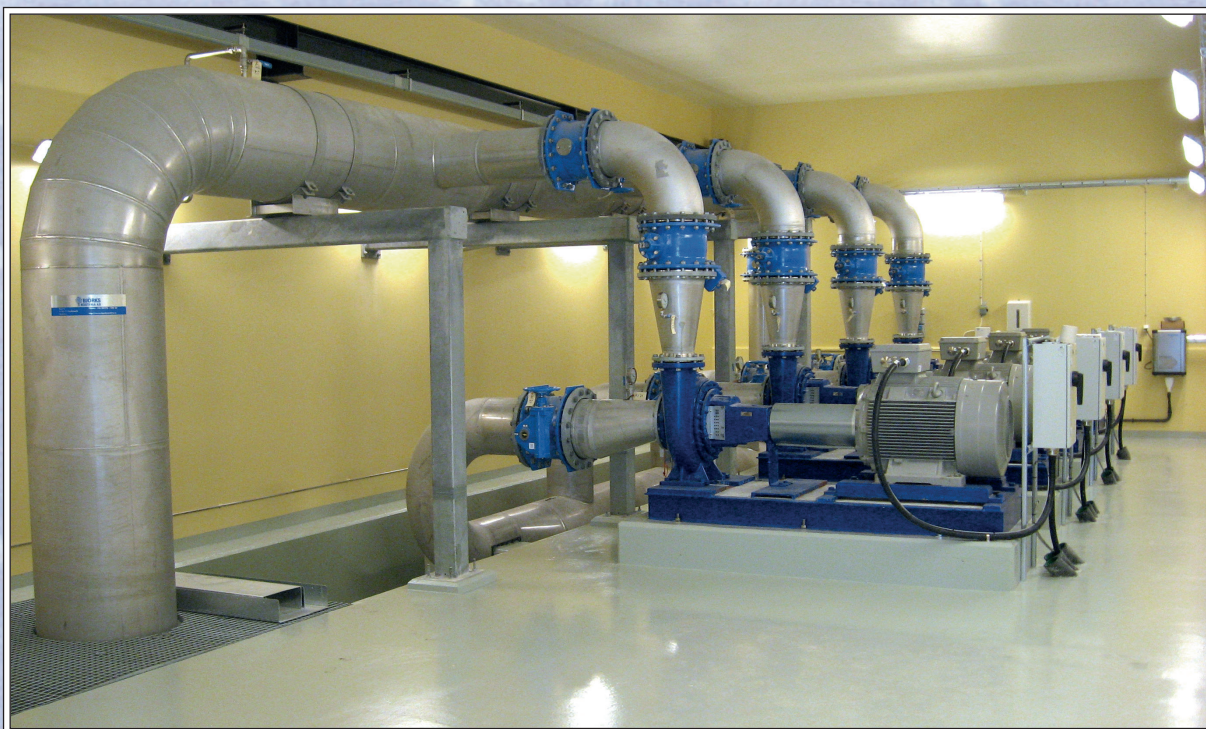
Pumpstation i drift.
